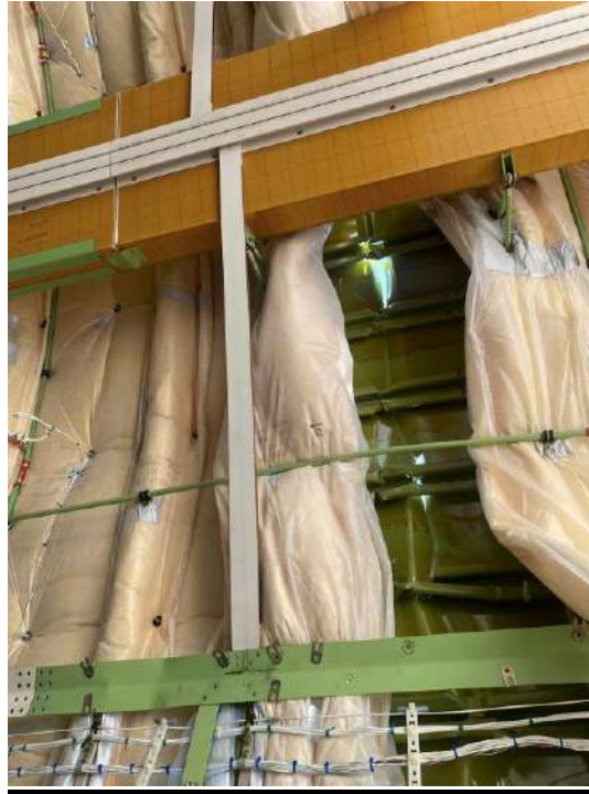
Figure 7: Upper crown fuselage damage as seen from the inside
